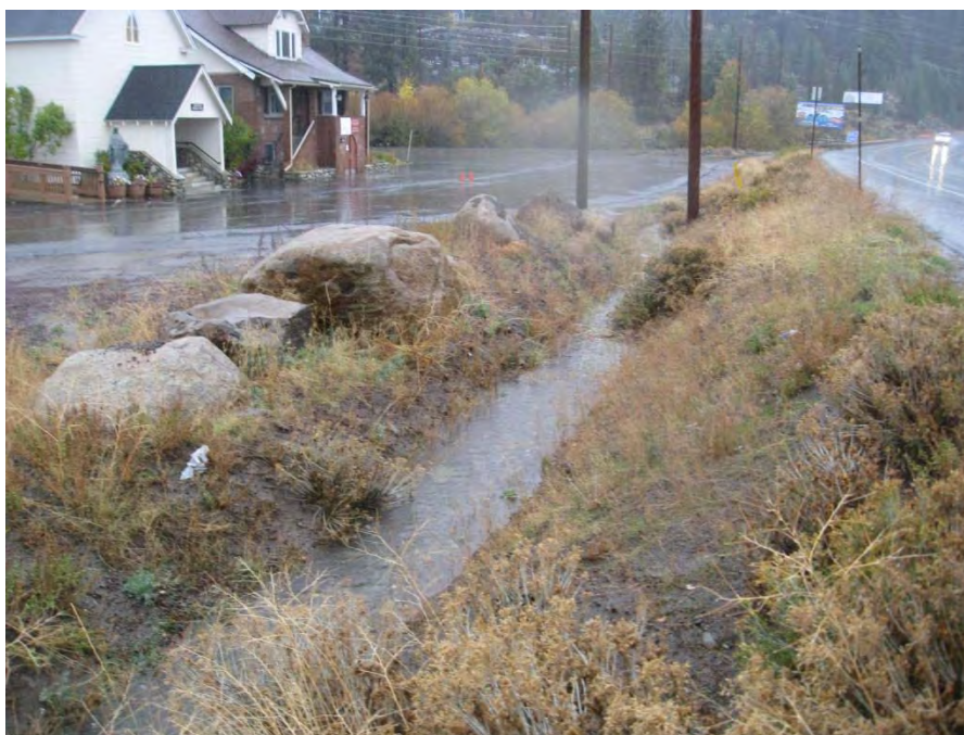
Figure 5-42 Vegetated Channel Draining Towards the Trout Creek SE Outfall (DSC-TC1)
