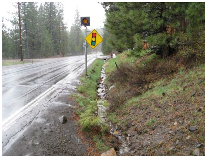
Figure 5-51 Earthen Channel Leading to the Donner Creek Outfall
