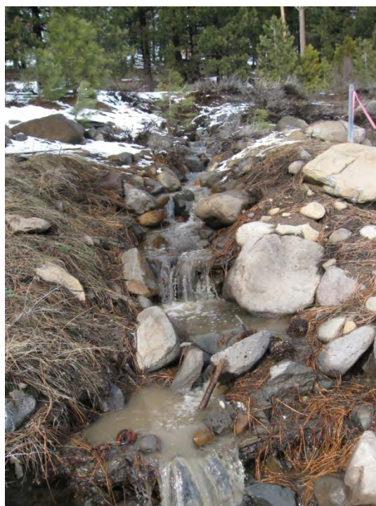
Figure 5-44 Steep Channel above Trout Creek NW Site
