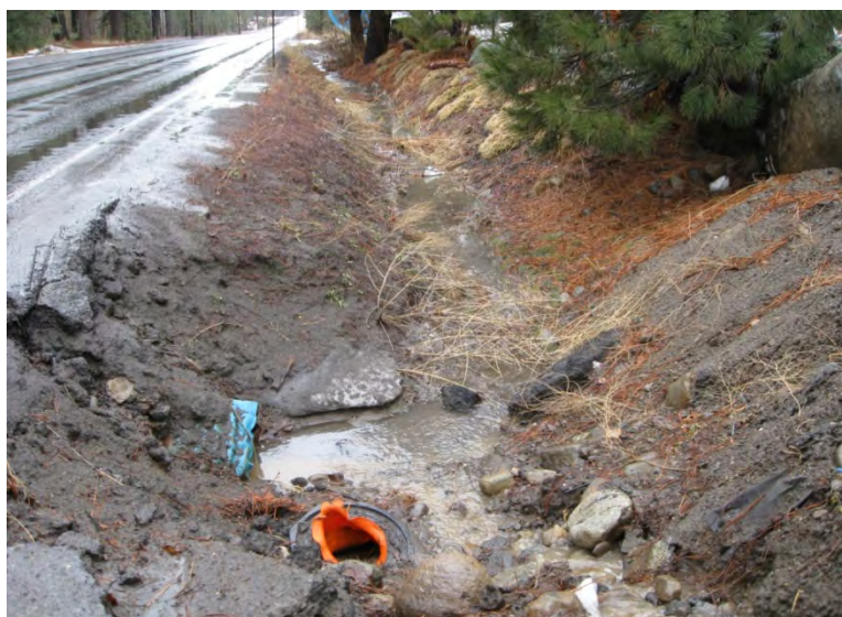
Figure 5-50 Earthen Channel Upstream of the West River Street Outfall (DSC-TT5)
