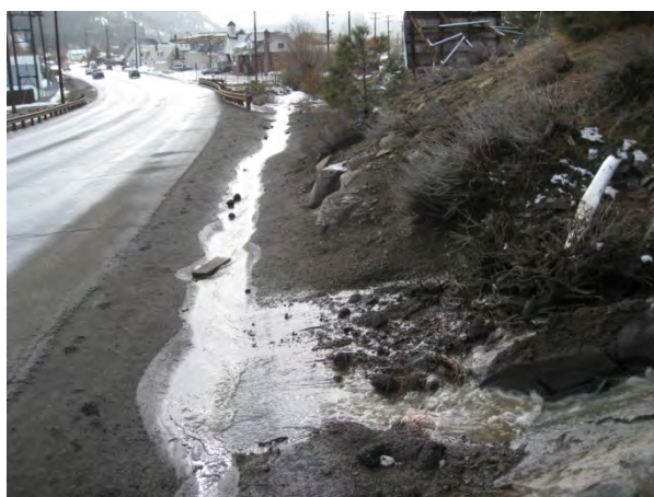
Figure 5-43 Asphalt Swale Leading to Trout Creek
