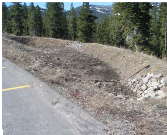
Figure 5-39 Infiltration/Sedimentation Basin at Northstar
