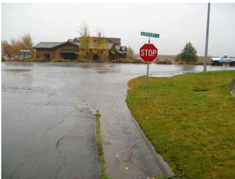
Figure 5-35 Airport Business Park Drainage Area on October 24, 2010
