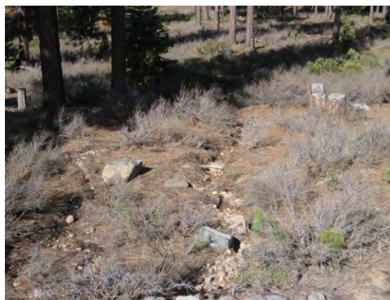
Figure 5-40 Erosion Downstream of Infiltration/Sedimentation Basin
